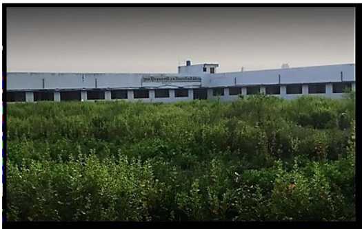
Figure 3 Old Building of School
